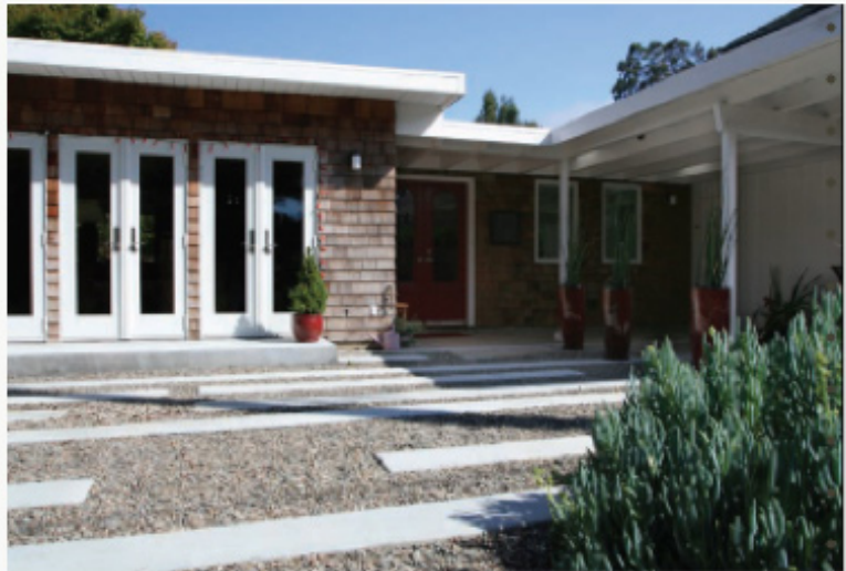
Permeable paving recharges the ground water and complements the lines of the architecture. Haughland shades of Green
